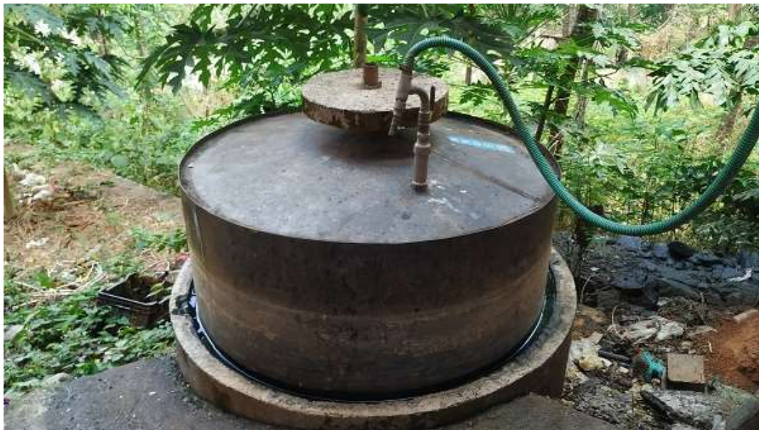
FIGURE 2: BIO GAS PLANT
